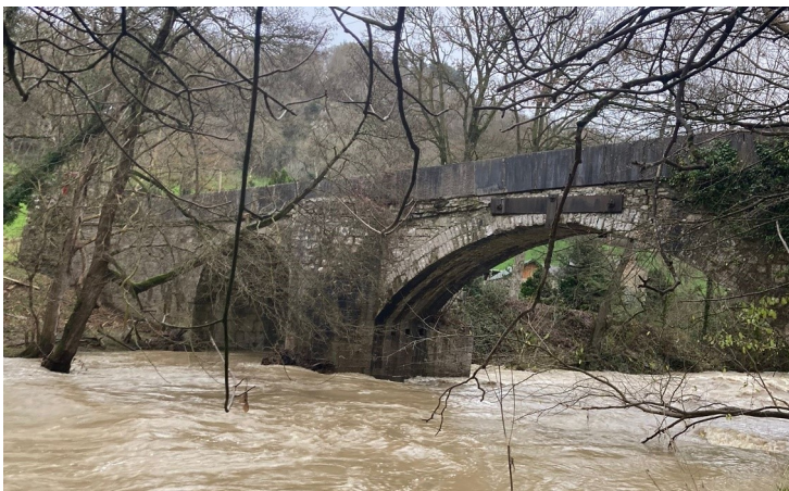
The bridge at Bontnewydd, with the River Elwy in full spate
